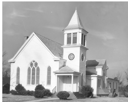
Church before Construction of Educational Building
