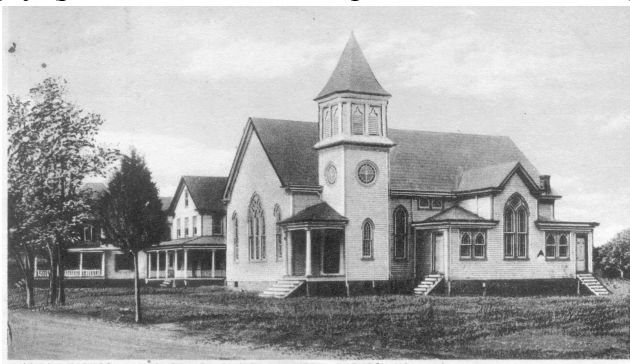
NEW KILMARNOCK BAPTIST CHURCH, CHURCH AVENUE, KILMARNOCK, VA.
